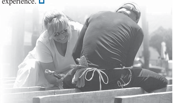
Castillo hard at work building houses in New Orleans with WAVNET.
